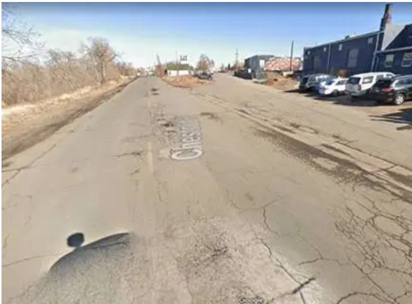
Arkins Court was a street used by RTD busses and the banks of the South Platte were a dumping ground. (Provided by Denver Parks & Recreation.)
